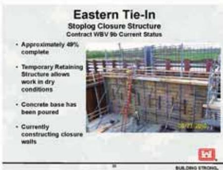
Now we are moving over to the Hero Canal and the closure structure, which has made huge progress in the last two weeks. We got the base slab in last Friday and we are now building walls. This is the slot right here that the stoplogs will be received in. We expect to pour these walls to elevation six this weekend. We will then go from elevation six to elevation 16 in the very near future. We will begin seeing a change in the Hero Canal with that closure structure.
