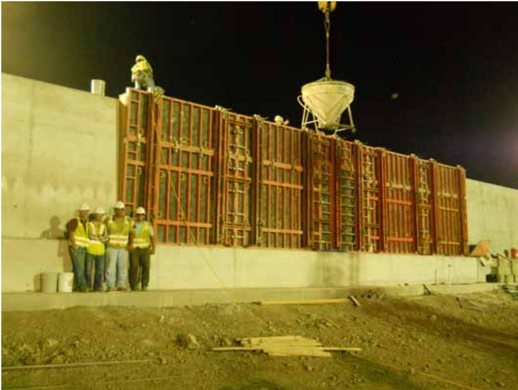
Image above: Cajun Constructors, Inc. completed the last concrete placement for contract LPV 148.02 late Friday night. The contract included construction of an eight-and-a-half-mile concrete floodwall from Verret to Caernarvon.
