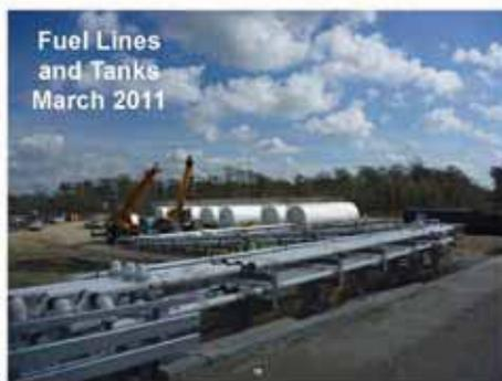
Here is a shot of the fuel tanks. They hold 300,000 gallons, enough to keep the pump station operating for three days continuously.
