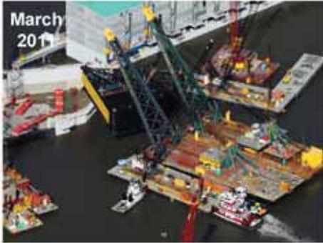
This is the placement of one of those large gates. It required two of Bisso's big heavy lift cranes that can lift 750 tons each.
