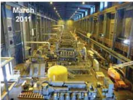
This is inside the pump station looking from the safe house. This is a shot of the engines and the driving pumps. They are 55-hundred horse power diesel engines.
